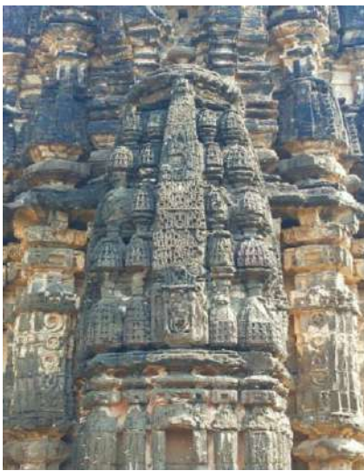
Figure 46 Miniature Shikhara as buttress
