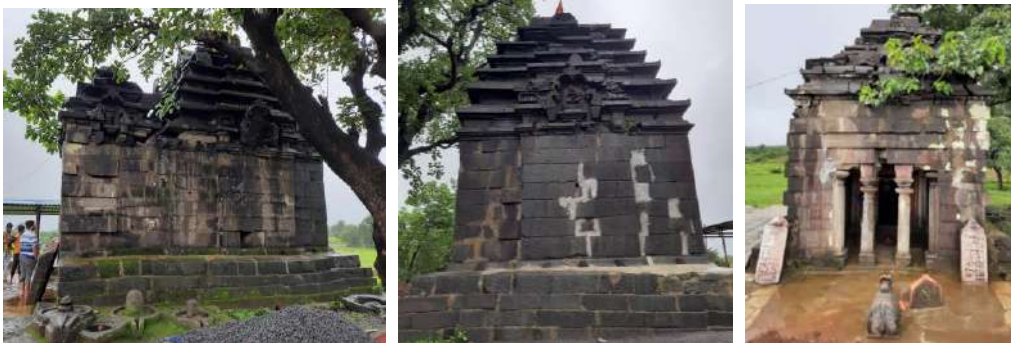
Figure 93: North façade, West façade, East facade
