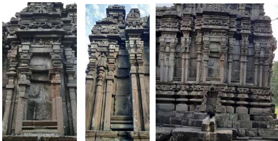
Figures 57 Façade details with Niches, Ardhastamba and northern façade of shrine
