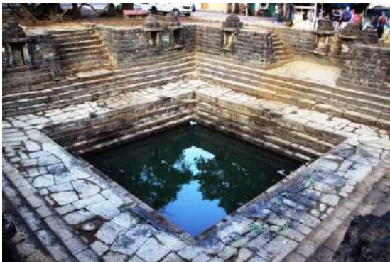
Figure 1: Pushkarni (Water tank)
