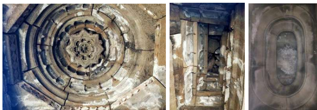
Figures 70,71,75 Domical ceiling, Vault ceiling, oval ceiling in temple 1
