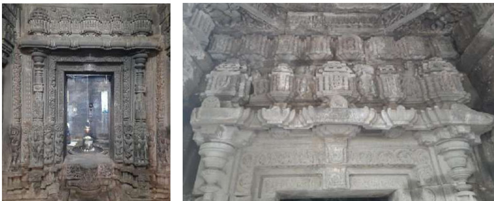
Figure 23,24: Doorway of main shrine, Lintel and cornice details
