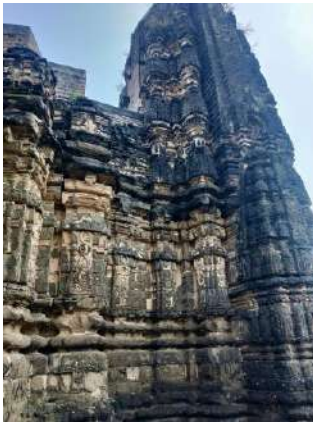
Figure 46 Miniature Shikhara as buttress
