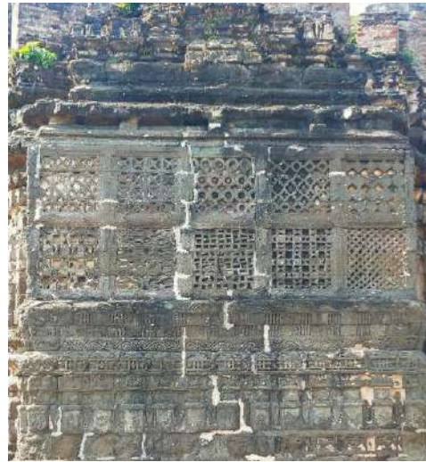
Figure 47 Closed porch cladded with jali pattern
