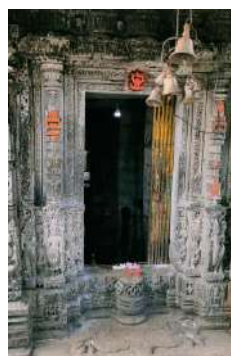
Figure 10,11: Door cornice and lintel detail, Eastern doorway & Western doorway
