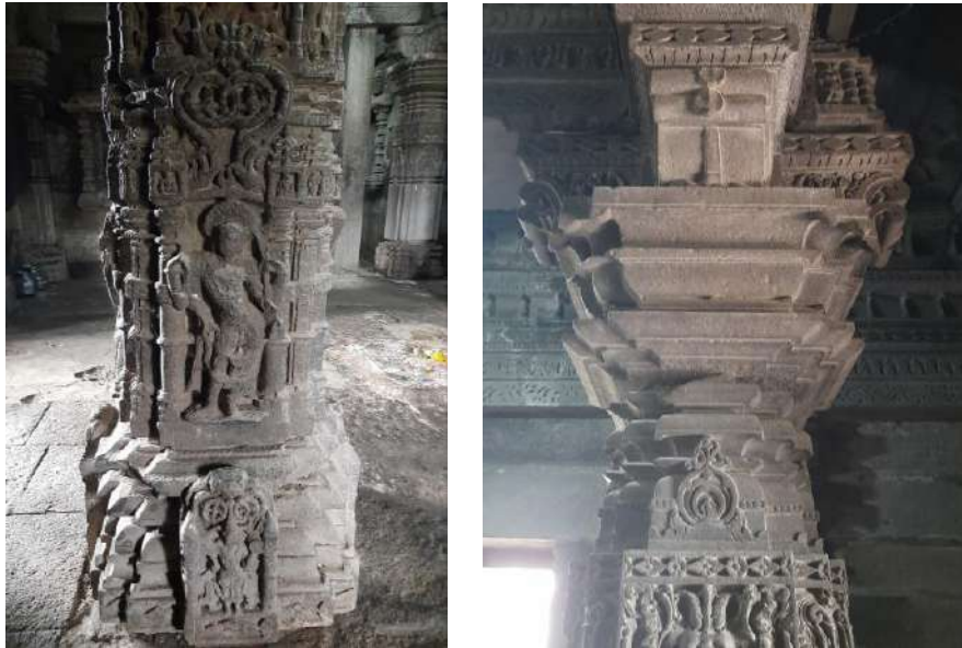
Figure 22: Rangamandapa columns detail, Base and Capital
