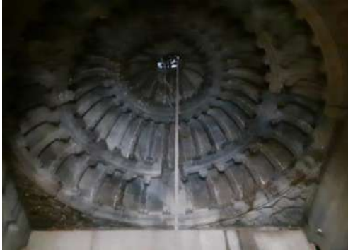
Figure 91: Domical ceiling in shrine
