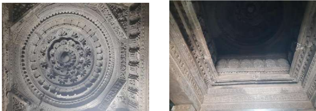
Figure 25,26: Domical ceiling over antarala , Domical ceiling over the rangamandapa .
