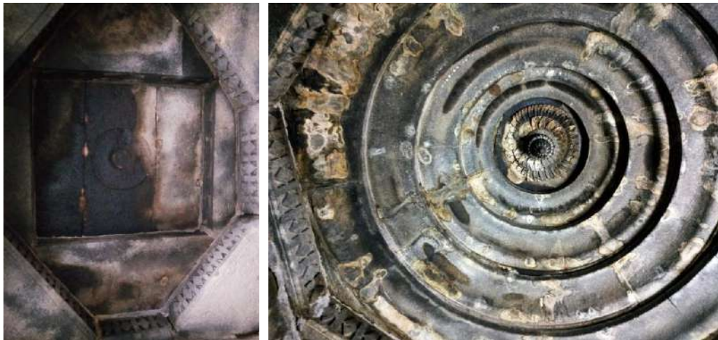
Figure 97 Box type ceiling and Domical ceiling
